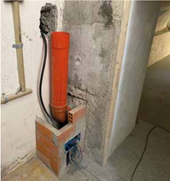
Preparation of extraction point
